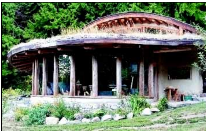
THE CHANNEL ROCK COB HOUSE is a grass-roofed cob house where students of Bainbridge Graduate Institute ( www.bgiedu.org ) meet for 11 intensives a year on Cortes Island. The rest of the work is done from home. — Photo Provided By Bainbridge Graduate Institute
