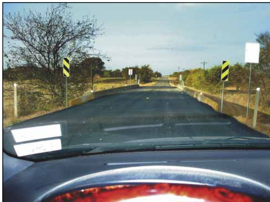
THIS TWO LANE ROAD has signs marking the bridge, but lack of sufficient lane width leave no room for error. Local say that this is a much greater concern than the trees.
