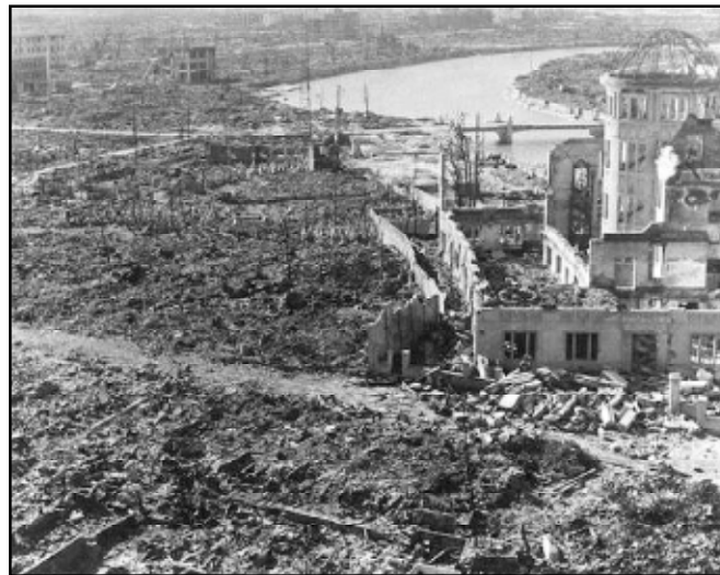
Hiroshima, Japan, the day after it was hit with a nuclear weapon. Notice the steel frame buildings that still stand, dotting the landscape.
