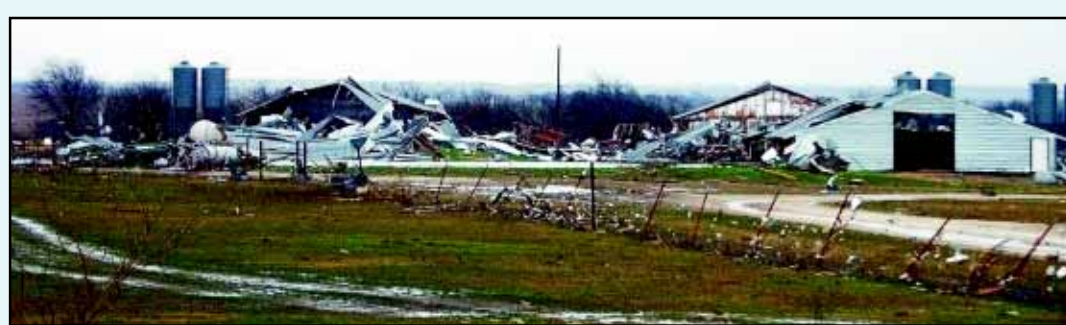
NOT MUCH LEFT — A turkey farm east of Clifton off of CR 708 and 3550 was nearly destroyed following Friday afternoon's tornado. The cell ripped through, laying fences down and demolishing barns.
